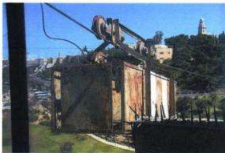
Solution to communication problem with Mount Zion posts (Photo: Ron Peled)
